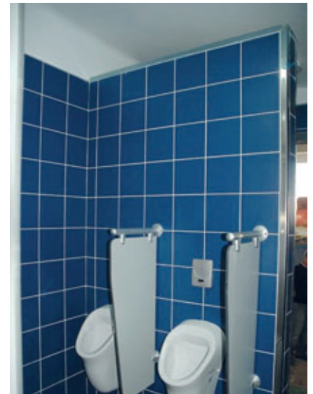
Fig. 4: The interior of a Precast Lavatory made in Turkey.
