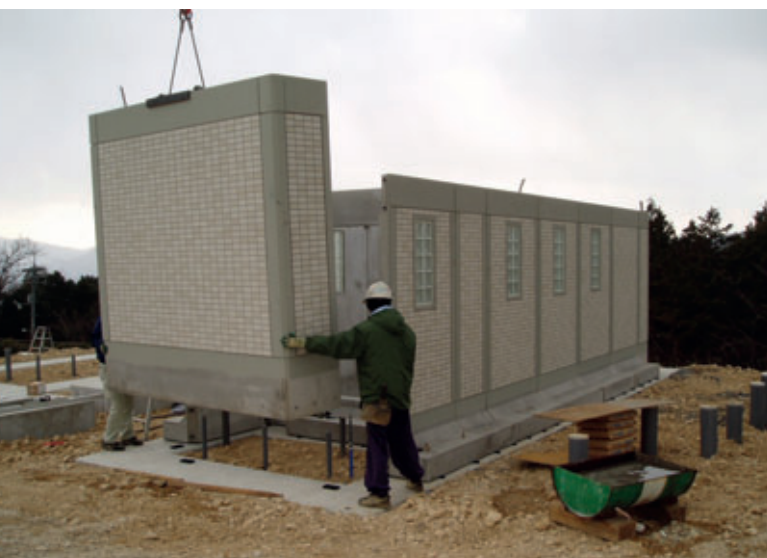
Fig. 2 and 3: Assembling the precast elements on construction site.
